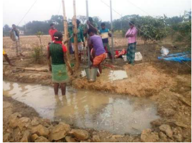
Fig.8.1. Pictorial view of installing observation well
